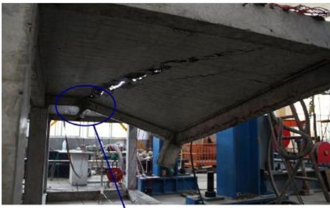
(a) Experimental Cracks for Slabs [21]
