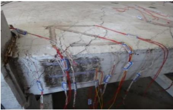
(a) Experimental Cracks of Beam (B) [20]
